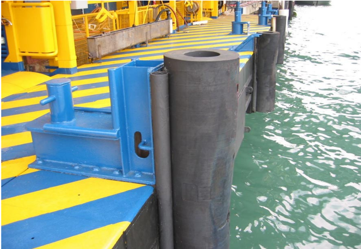
Plate 5 – Cylindrical Fenders
